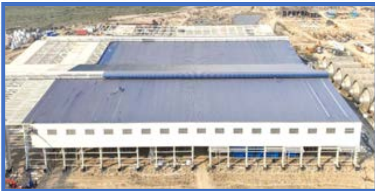
Os&Us Area – PVC Bagging Warehouse
