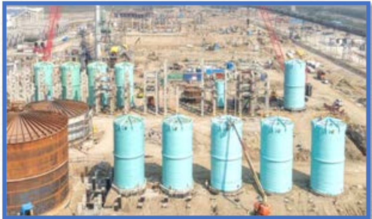
Os&Us Area – Non Metallic Tank Erection
