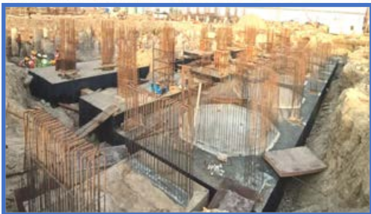
Chlor - Alkali Plant - Waste Gas Treatment
