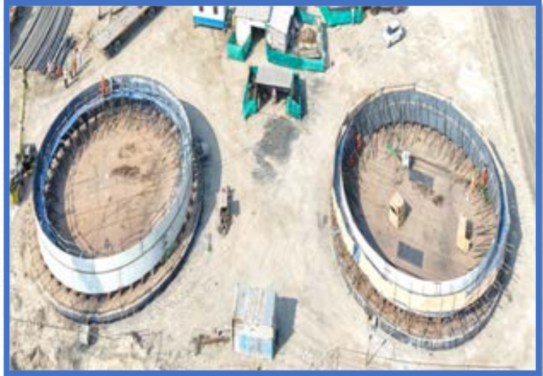
Acetylene Plant Gas Holder
