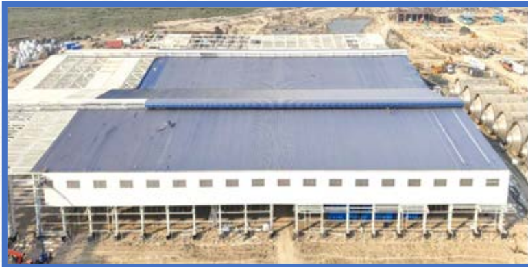
Os&Us Area – PVC Bagging Warehouse
