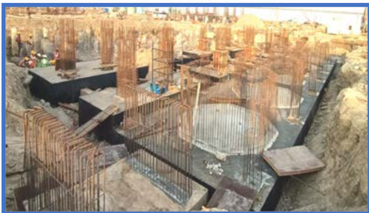
Chlor – Alkali Plant – Waste Gas Treatment
