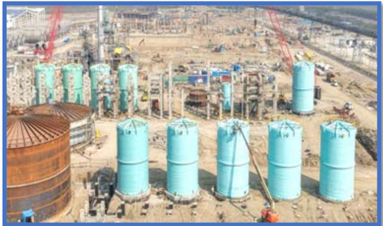
Os&Us Area – Non Metallic Tank Erection
