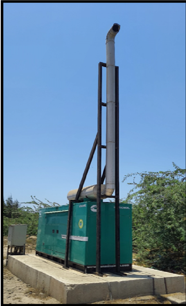
D.G. Sets having adequate stake height and Acoustic system covered on it.
