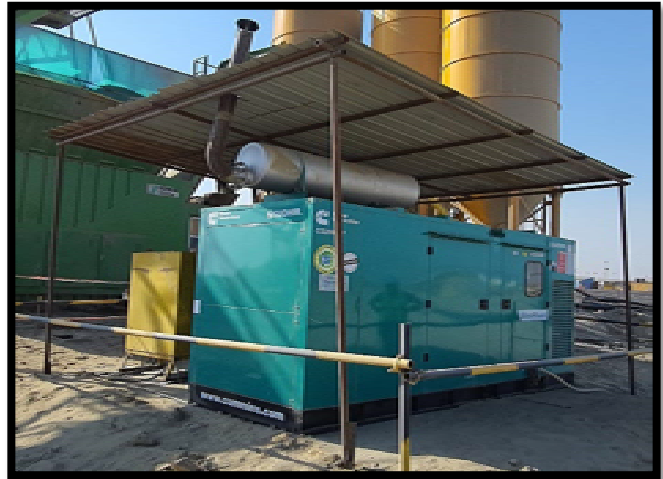
D.G. Sets having adequate stake height and Acoustic system covered on it.
