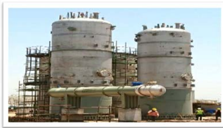
PVC Plant - Equipment Erection
