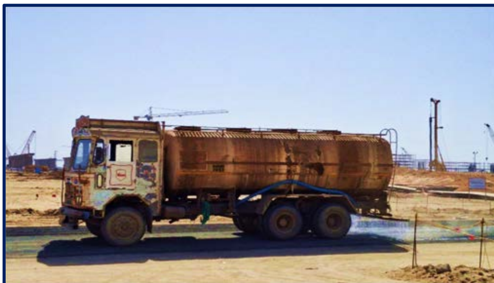
Water Sprinkling on Internal Roads
