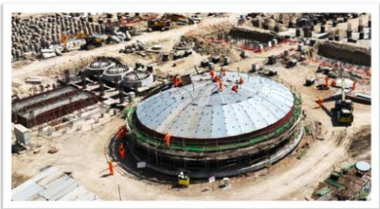
VCM Gas Holder – Tankage Erection Work – PVC Plant
