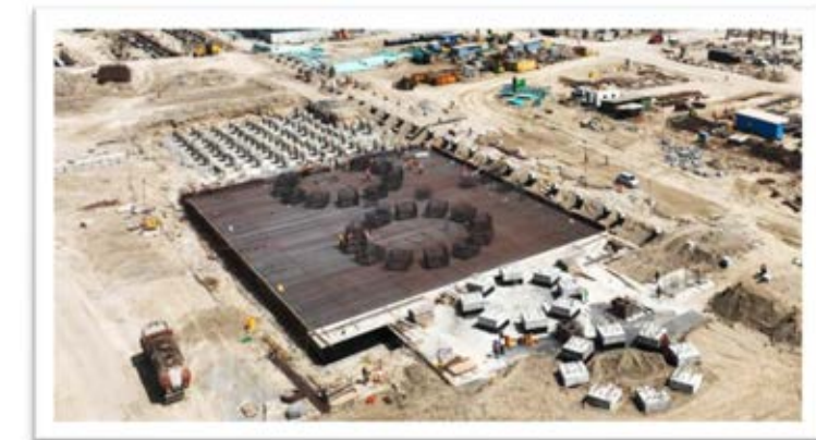
VCM Sphere – RCC Sub Structure Work
