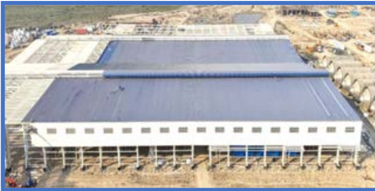
Os&Us Area – PVC Bagging Warehouse
