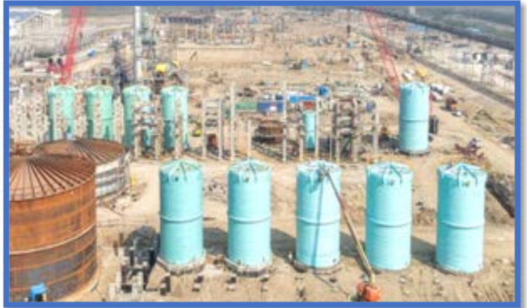
Os&Us Area – Non Metallic Tank Erection
