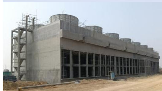
Induced Draft Cooling Tower
