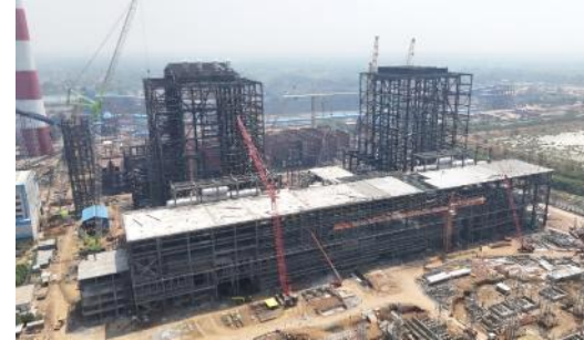
Unit #2 Electrostatic Precipitator
