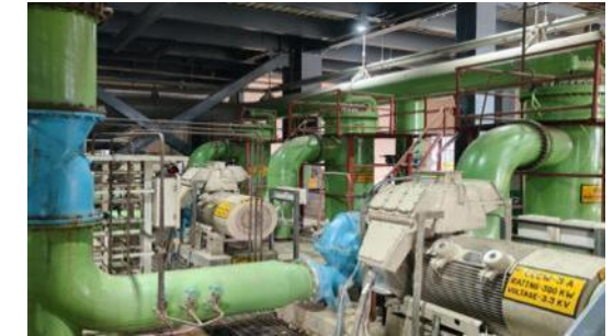
Circulating Water Motor Erection
