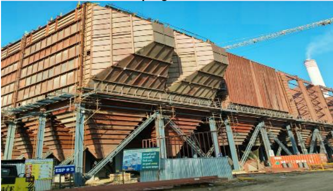
Unit #3 Electrostatic Precipitator Hopper erection work progress
