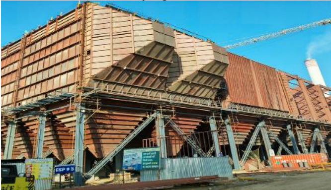
Unit #3 Electrostatic Precipitator Hopper erection work progress
