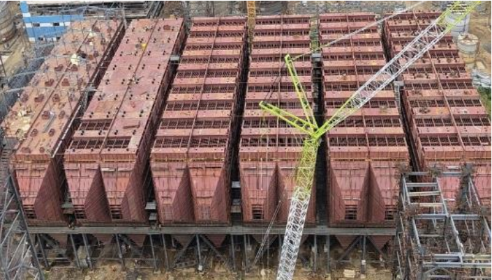
Unit #4 Electrostatic Precipitator
