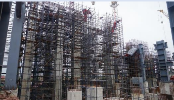
Unit #2 Turbine Generator Deck Column Casting
